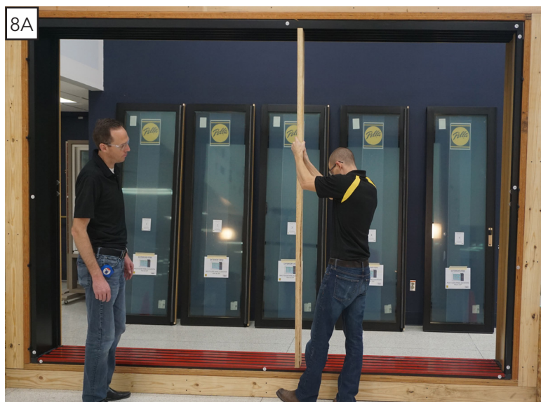
Measuring for gauge board
