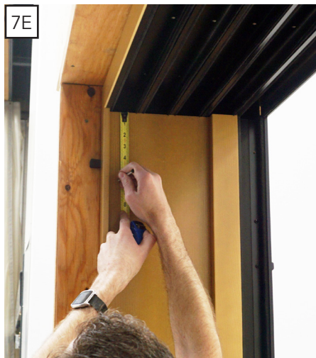
Marking for pilot hole location
