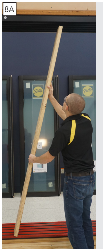
Positioning gauge board
