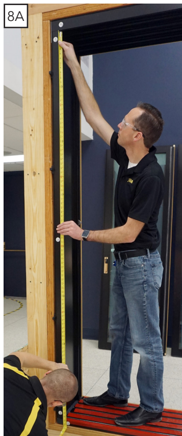
Measuring for gauge board
