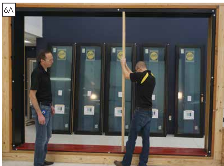
Measuring for gauge board
