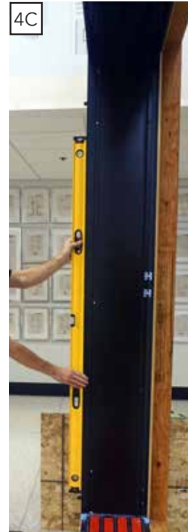
Use level to check plumb of frame to confirm frame is straight up and down in the opening.
