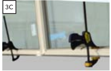
Stiffener bar clamped to subassembly
