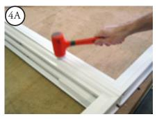
B. **Center the wooden reinforcement** along the length of the mullion to achieve an equal set-back from the each end of the mullion.
