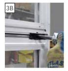
C. Install the mullion cover. Use a mallet to seat the cover into the window accessory grooves.
