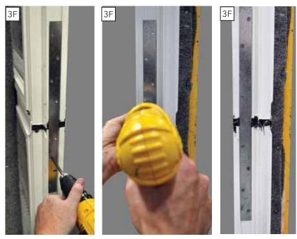
G. Apply two 6"-8" pieces of flashing tape over the sealant and end clip on each end of the mullion. Start one piece of tape flush with the exterior edge of the frames and overlap the clip. Start the other piece of tape flush with the interior edge of the frames and overlap the clip.
