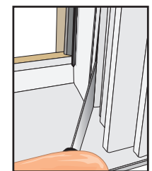
Pry off Monumental Double-Hung jamb liner
