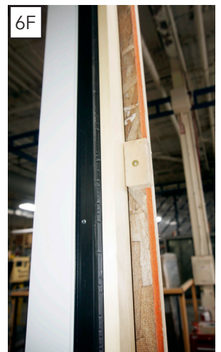
Frame positioned against block from 6D.
