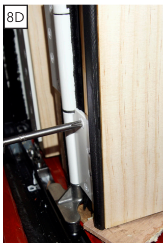
Attaching bottom carrier hinge on second panel
