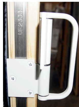
Attaching Middle Hinge with Handle Pull
