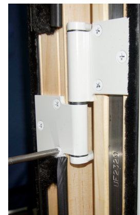
Attaching Middle Hinge with Handle Pull
