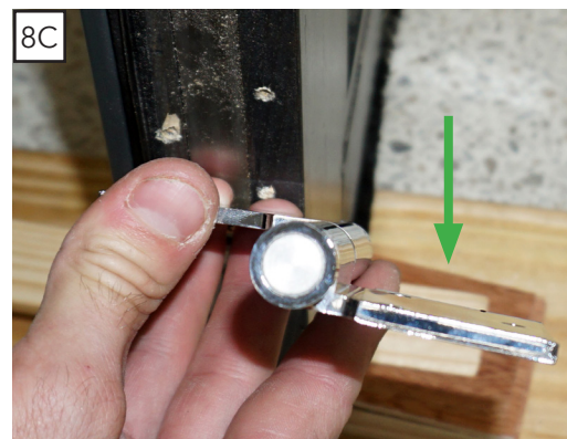
Top View showing correct off-set hinge orientation from Left Jamb
