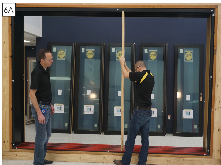
Measuring for gauge board
