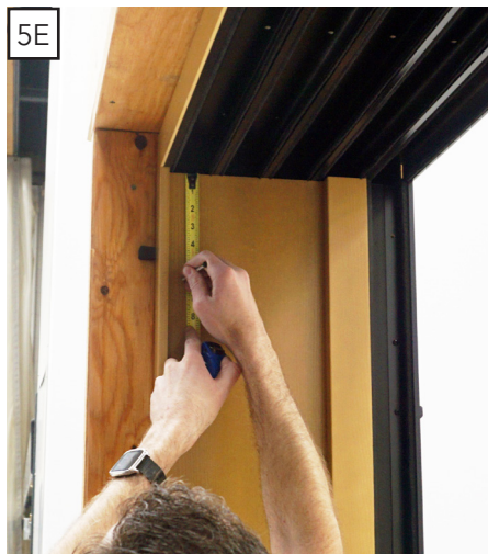
Marking for pilot hole location
