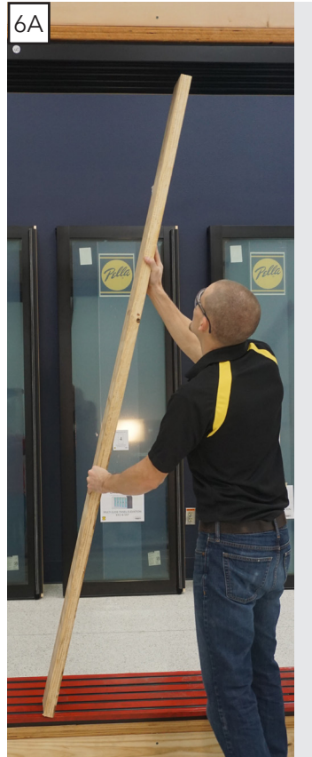
Positioning gauge board
