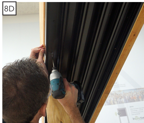
Frame Installation Screw
