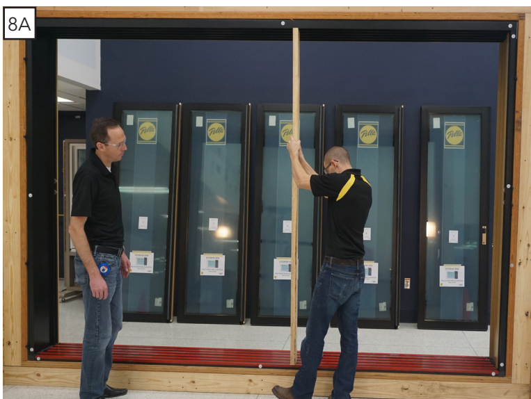
Measuring for gauge board
