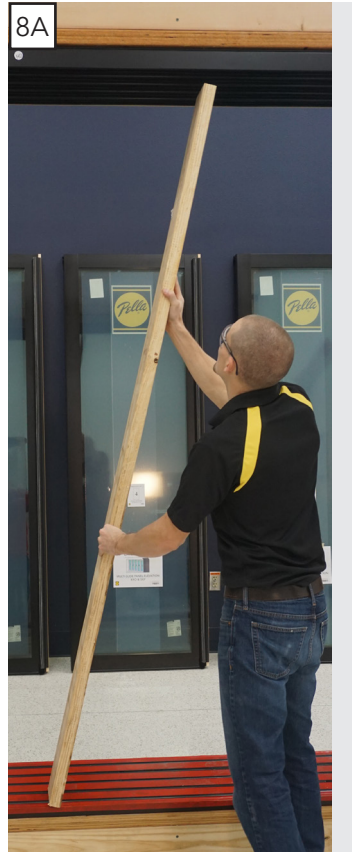
Positioning gauge board
