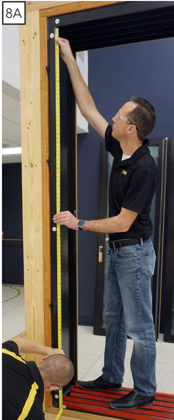
Measuring for gauge board
