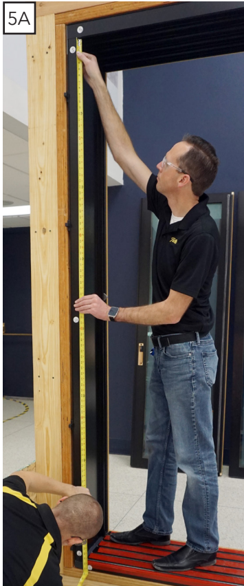
Measuring for gauge board
