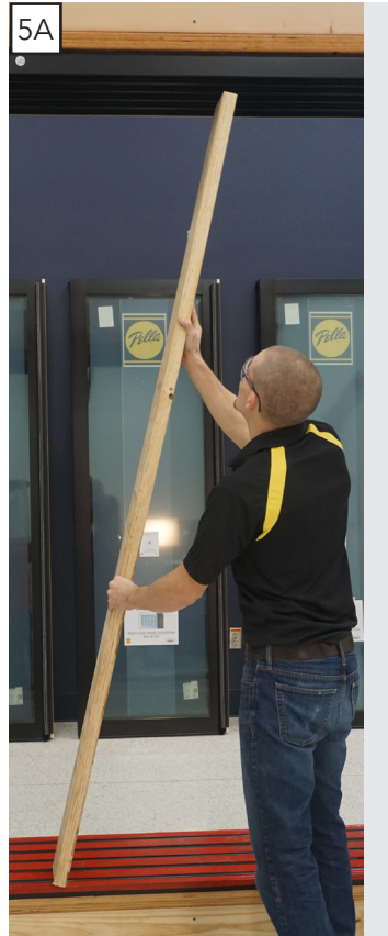
Positioning gauge board
