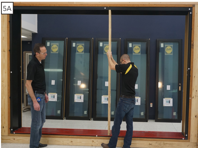
Measuring for gauge board
