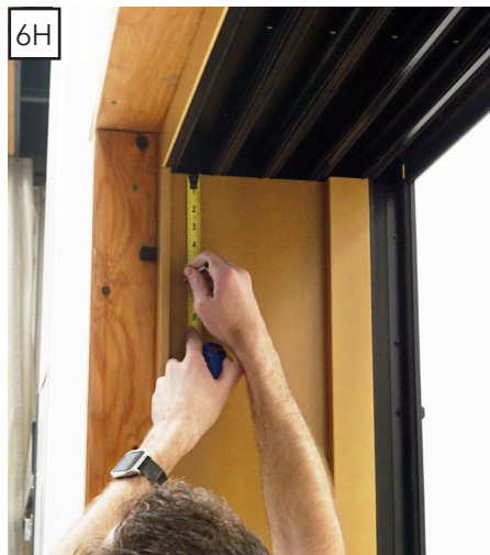
Marking for pilot hole location
