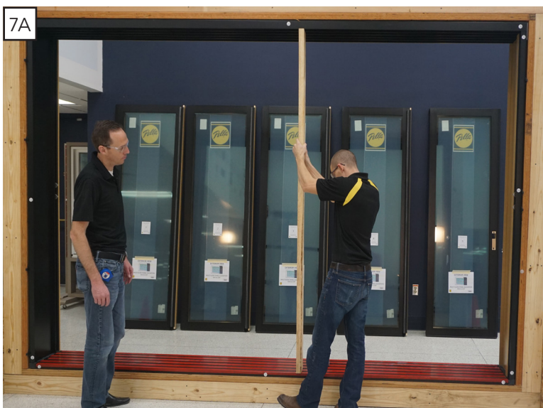
Measuring for gauge board
