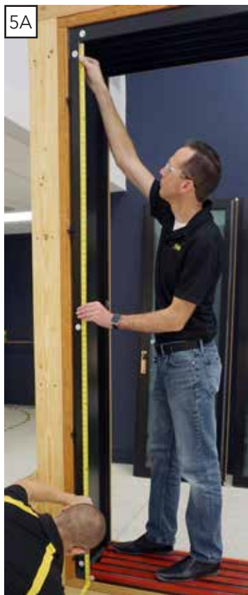
Measuring for gauge board
