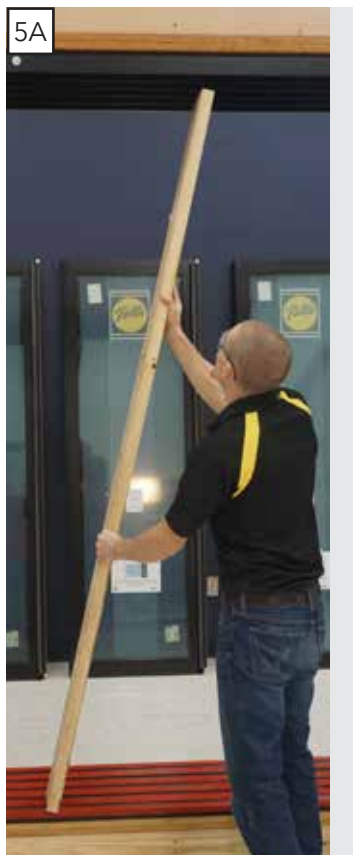
Positioning gauge board
