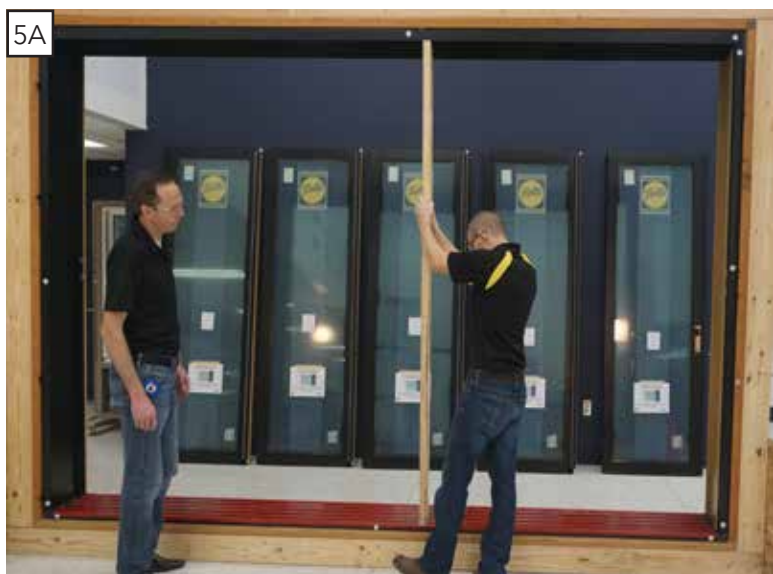
Measuring for gauge board
