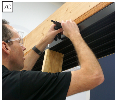
Frame Installation Screw
