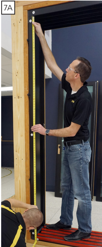
Measuring for gauge board
