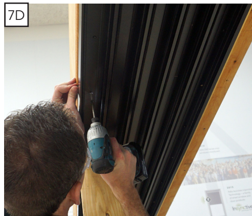
Frame Installation Screw
