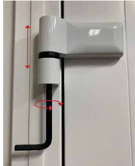
Up and down adjustments: adjust ALL hinges evenly to distribute the weight evenly.
