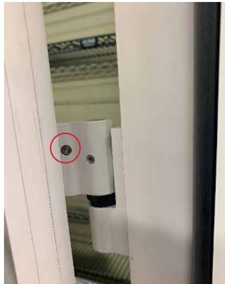
Back out set screw to remove face plate.
