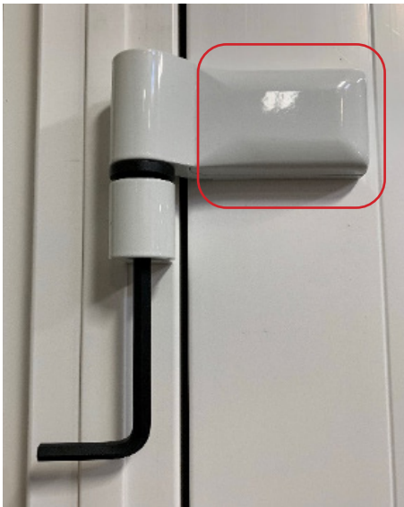
Remove hinge cap for side-to-side adjustments.
