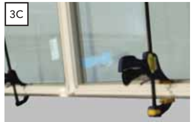
Stiffener bar clamped to subassembly
