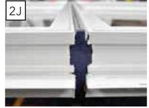
K. Place 4 six inch (6") lines of sealant on each end of the mullion. One line of sealant goes on each side of the mullion reinforcement and one in each of the window accessory grooves.
