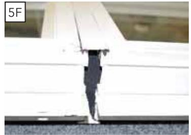
G. **Fill each end of the mullion with sealant.** On Horizontal mullions completely fill each end with sealant. **Vertical Mullions only:** Leave a 1/4" gap in the sealant on the exterior side at the bottom only to act as a weep for the mullion joint.
