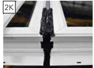
L. Install the mullion cover. Use a mallet to seat the cover into the window accessory grooves. Clamps may also be used to help draw the mullion joint together.
