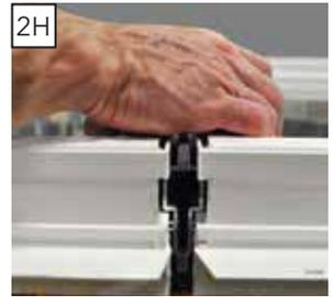
**Note:** Clamps may be used to help draw the windows together and ensure adequate tape adhesion.
