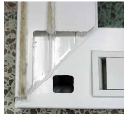
Interior view - bottom corner of interlocker panel
